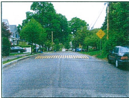
Temporary Speed Hump
