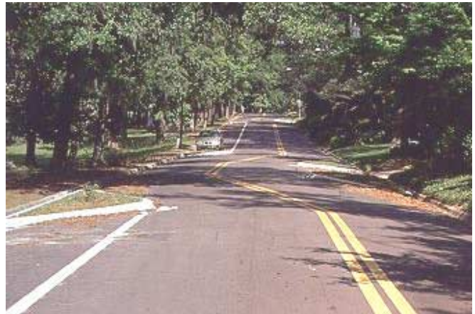
Islands are placed in this roadway to create a chicane, forcing traffic to slow down for the lateral roadway shift. Source: Batson
