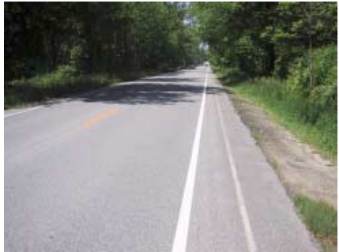
On this New York State roadway just west of Ridgefield, CT the travel lane has been narrowed from 12 to 10 feet.
