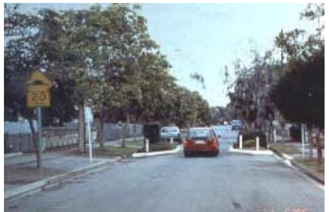
Two islands are placed directly opposite one another, allowing only one vehicle to pass at a time. Source: TrafficCalming.Org
